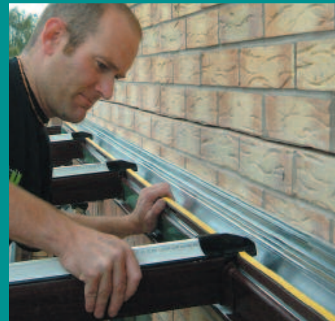
Glazing bars just click into place
